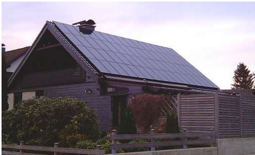
15kwp Sunpower „fullblack“ (2011)
